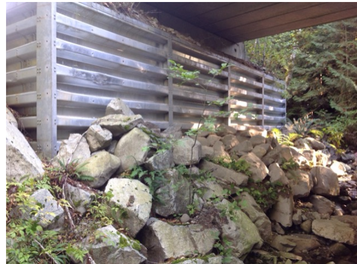
Right Bank Abutment when facing downstream
