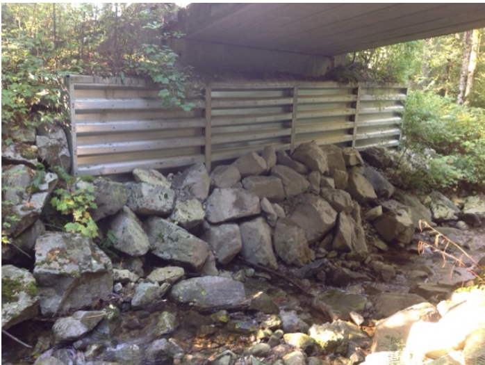
Left Bank Abutment when facing downstream
