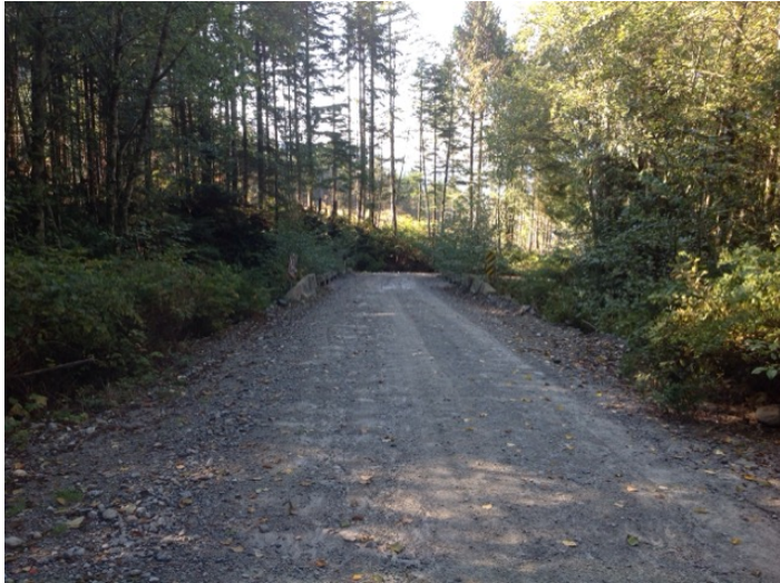
Approach from Right Bank when facing downstream
