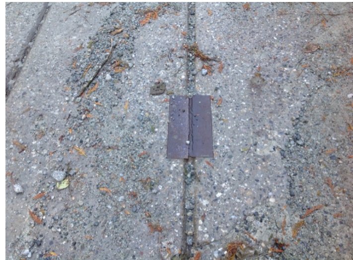
welded shear keys
